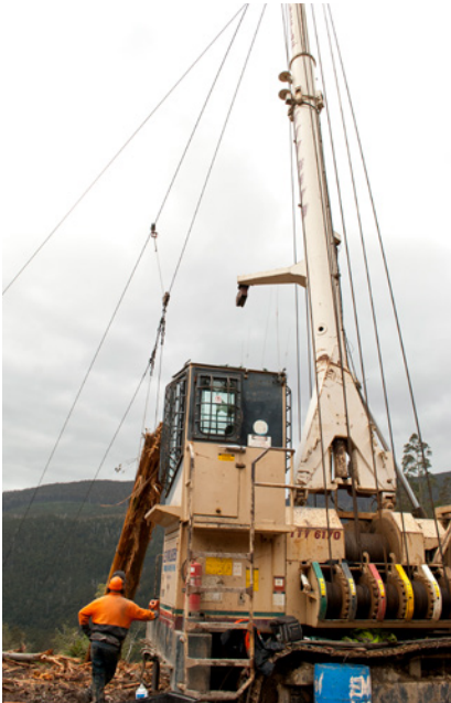
Cable harvesting tower showing guy ropes.
