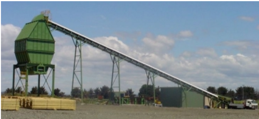
Plate 10 Typical Overhead wood fibre bin
