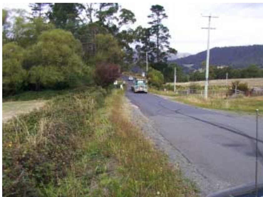
Truck over one lane Bridge North Huon Rd.
