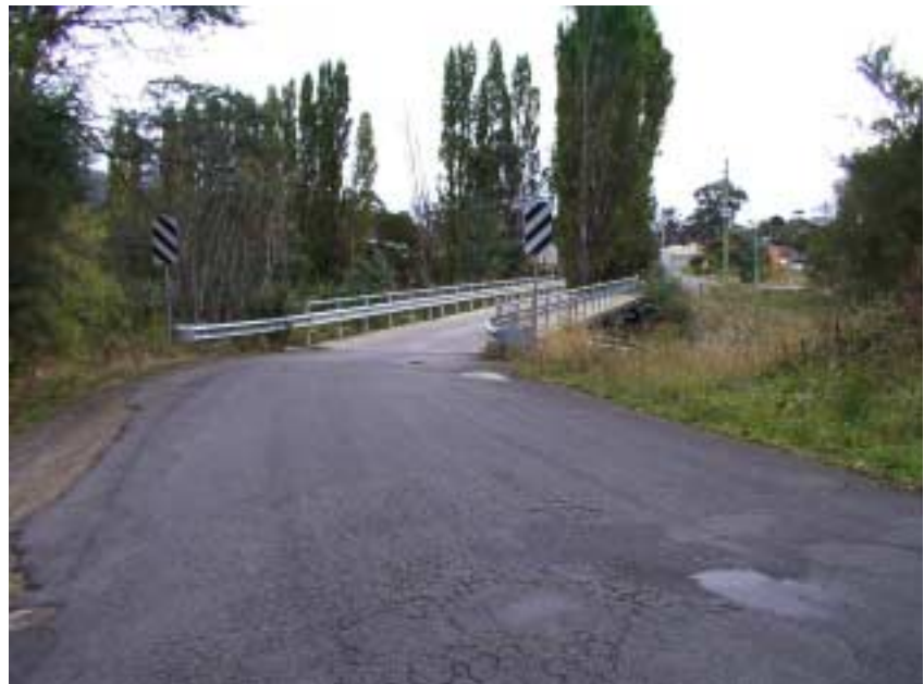
Mountain River Bridge one lane
