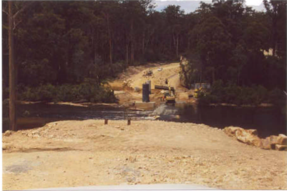
Construction of bridge across Huon River. Disused Quarry.
