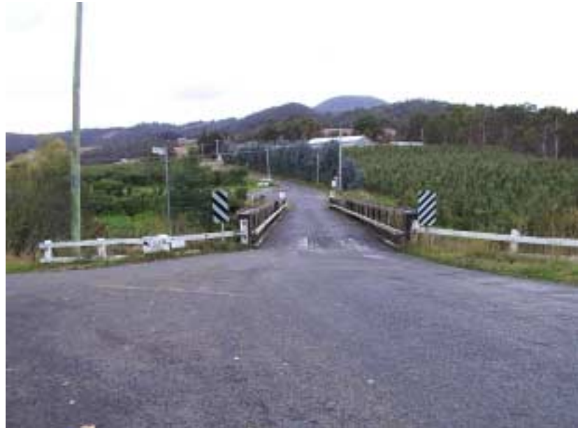
Mountain River Bridge Lollara Rd.
