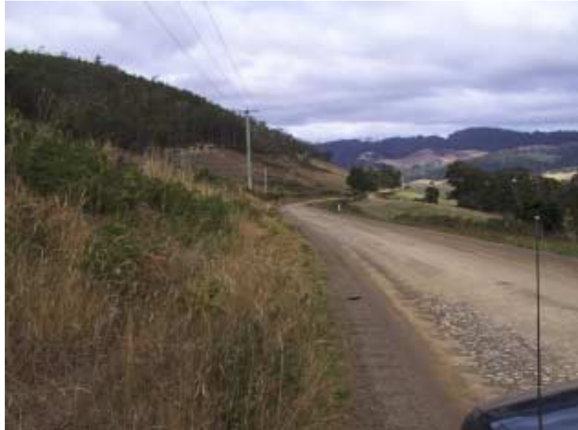
Gravel formation North Huon Rd.
