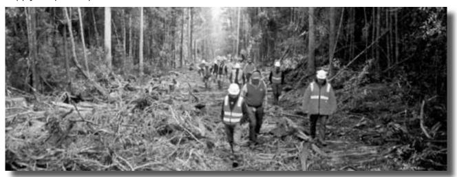
Figure 2. Primary snig tracks were cleared to a minimum width of about 9 m to allow an excavator to rotate at least 180 degrees. Slash was piled onto the cleared area to protect the soil and make a semi-permanent extraction path.
