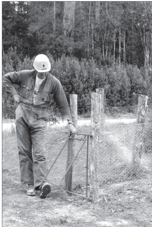
A fenced blackwood regeneration area with a ‘Blakey’s’ one-way wallaby gate, 2005. These gates (an innovation developed by Kevin Blake in the Smithton, now Murchison, District) allowed browsing animals trapped inside the regeneration area to escape through the one-way swing gate built into the corners of the fence. (Leigh Edwards demonstrates the gate’s operation.)
