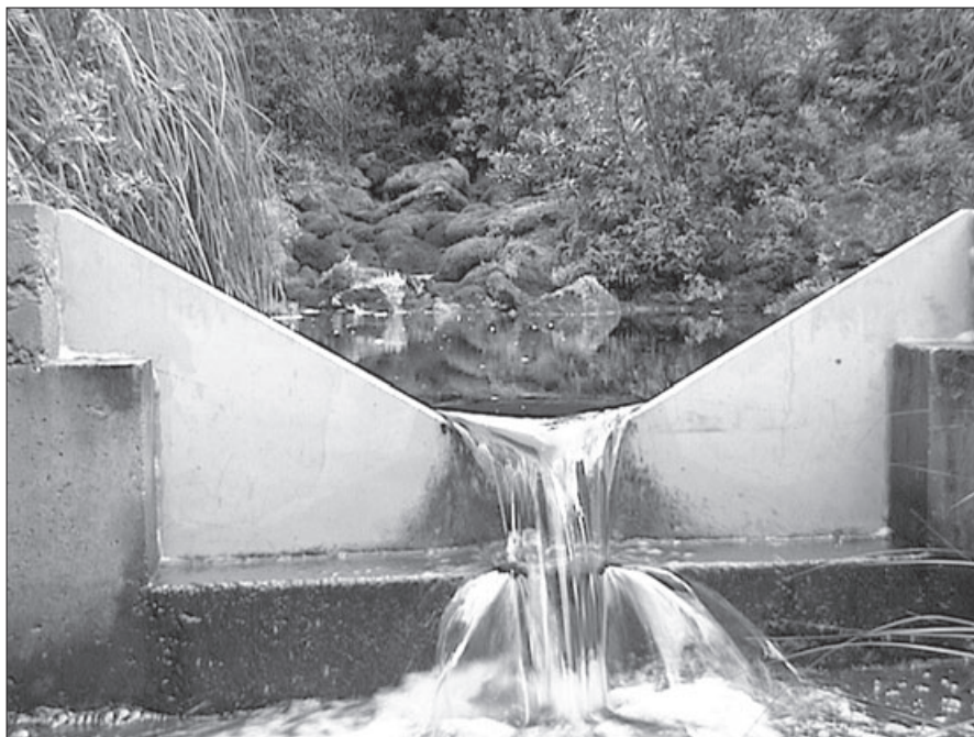
The weir on Swanson Creek in the Warra LTER Site.
