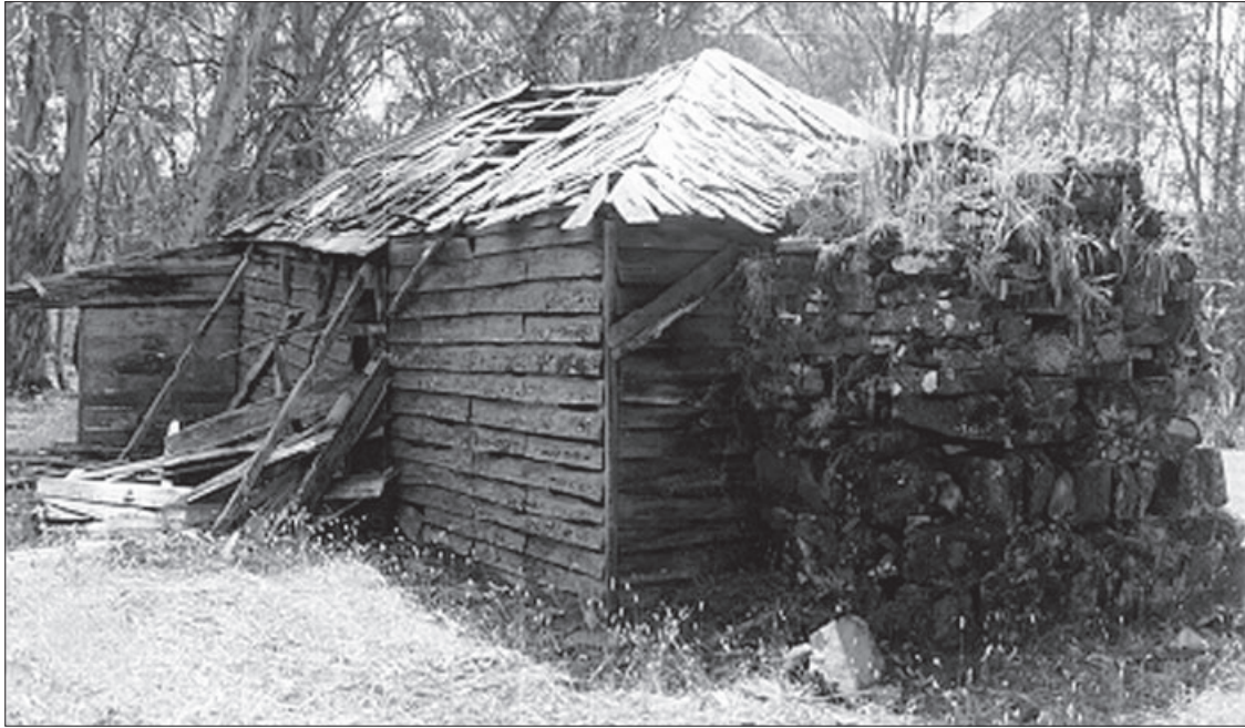
An abandoned shepherd's hut in the southern Central Highlands, one of the sites recorded in the Historic Sites Inventory Project in the 1990s.
