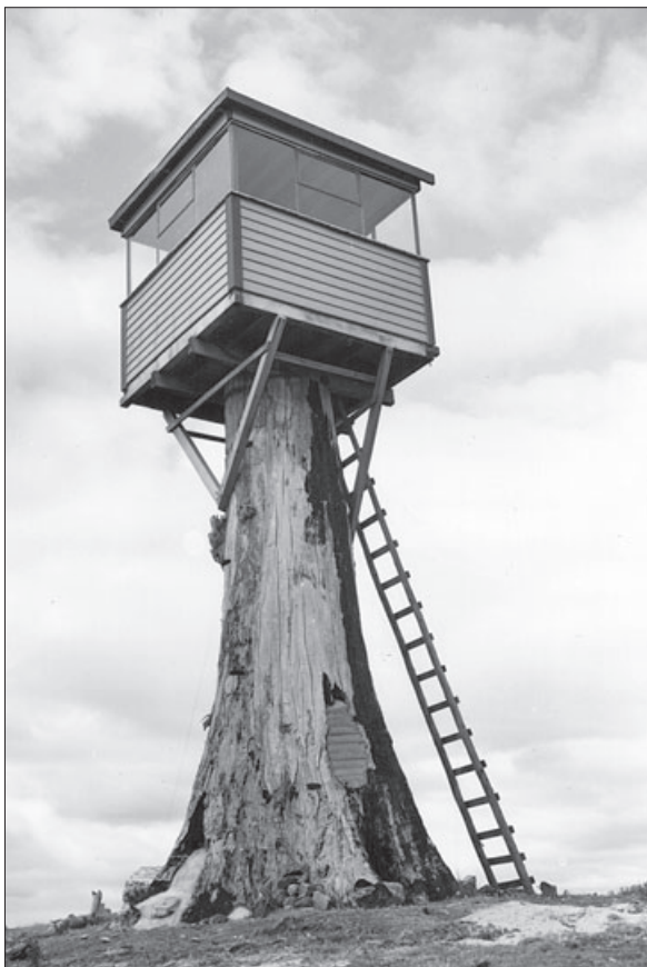
An early fire tower at Walduck Hill, south of Scottsdale in north-eastern Tasmania, 1950.
