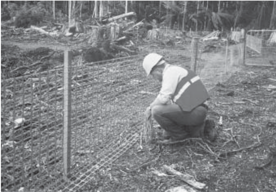
Photo 2. Pegging down the bottom of the barrier mesh.
