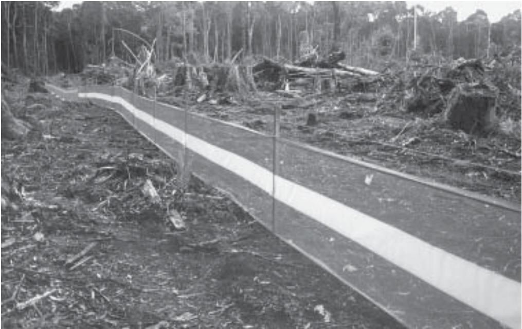
Photo 1. A section of onion bag mesh attached to top and bottom wires.
