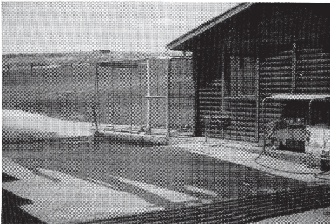
Fig. 3. Vehicle bath, pedestrian footbath and steam cleaning unit installed at Perth Nursery (Native Point).
