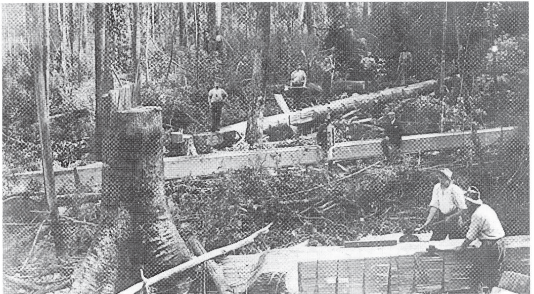
Photo 1. Hand hewing blue gum beams in the Southern Forests. (Courtesy: Forestry Commission, Tasmania)
