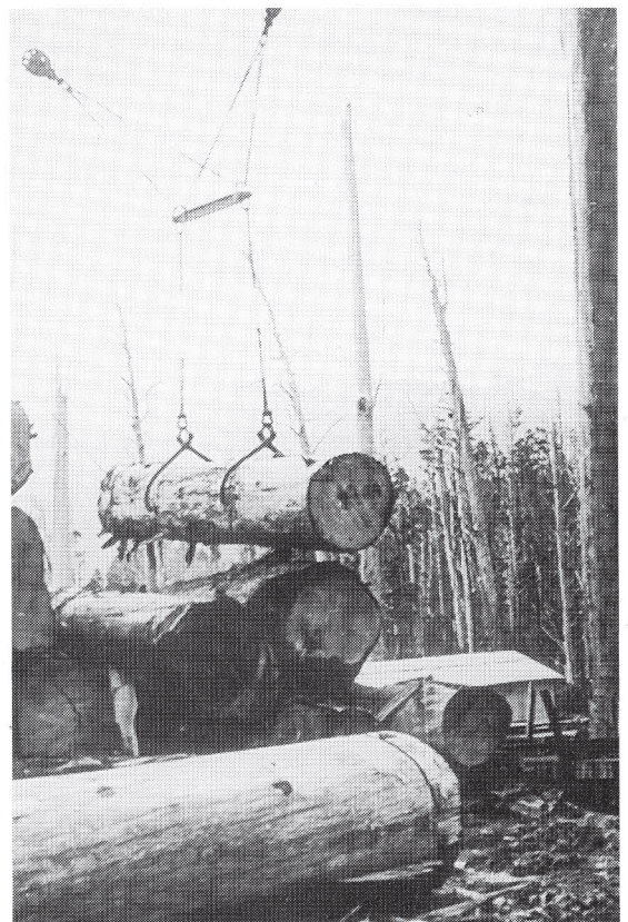
Photo 7. Loading with an overhead cable system. (Courtesy: Australian Newsprint Mills Ltd)
