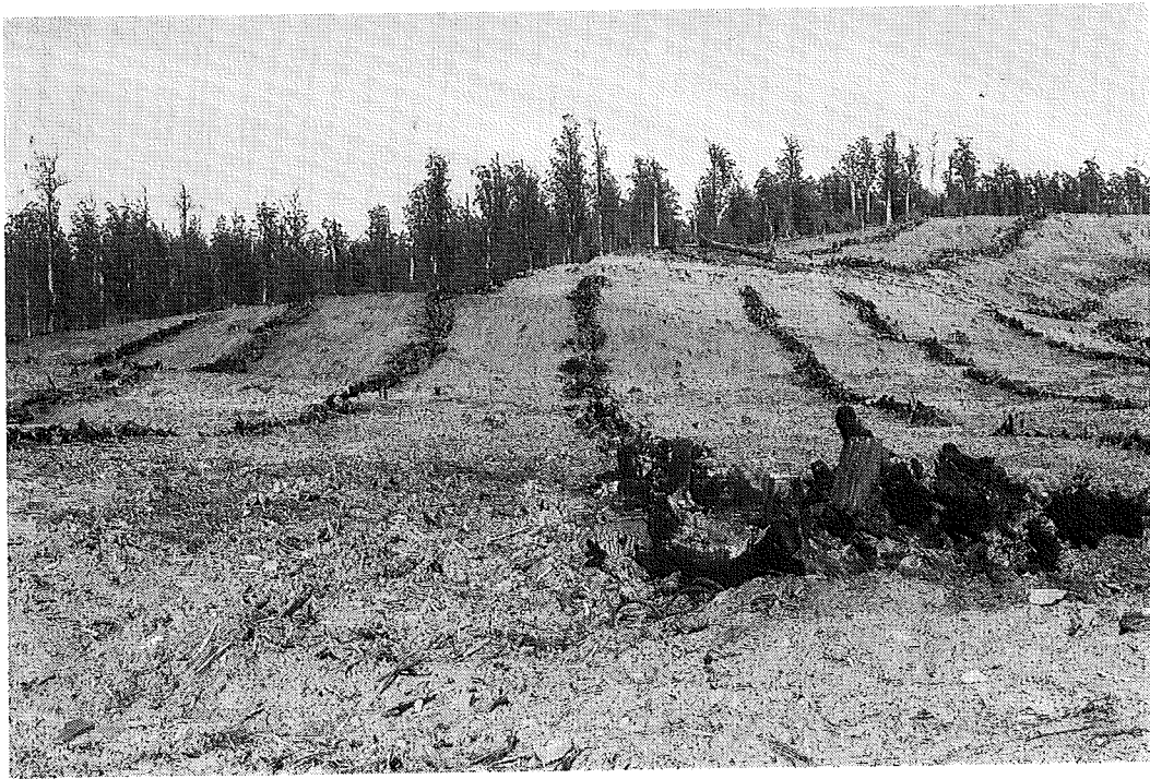
Photo 2. Windrows (above) pushed by bulldozer at Arve B, and (below) stacked by excavator at Arve X, after burning.
