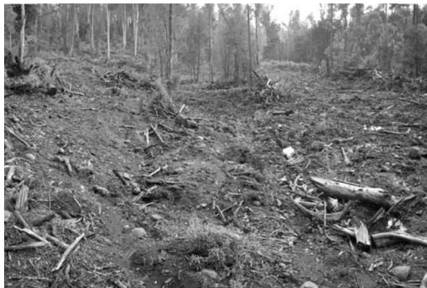
Photo 4. After machine scarification.
